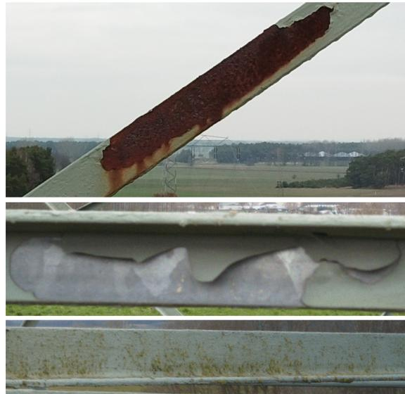
Figure 1: Examples of a corrosion damage, a missing painting damage and a patch of dirt, from top to bottom.
