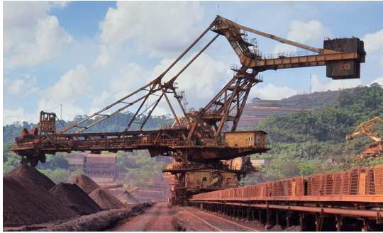
Figure 12: Bucket reclaimer used for field tests.
