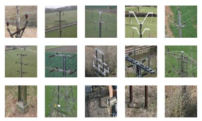
Figure 1: Top: images of S-type towers. Middle: images of T-type towers. Bottom: images from which tower type is not apparent.
