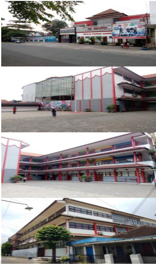
Figure 1. Existing Condition of Nasima Elementary School
