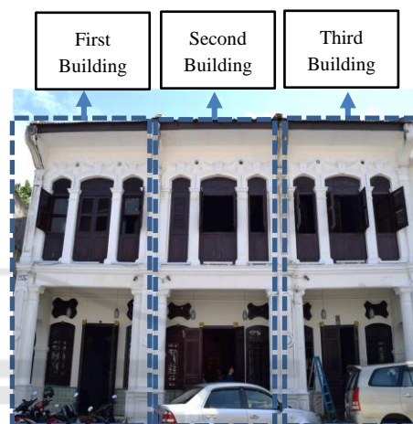
Figure 3: The Façade of the Traditional Courtyard Shophouses No.3, 5, 7. Source: Field Work
