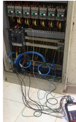
Figure 5: Installation of combined power measurement.
