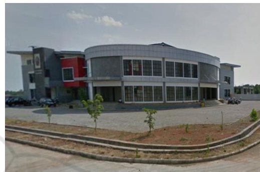
Figure 2: Electrical department building from left side.
