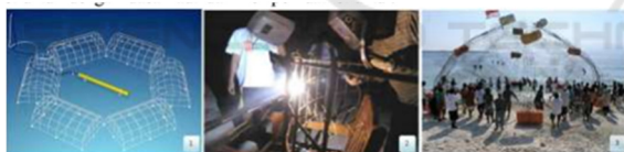
Figure 1: The making of biorock structure ( https://monruw.wordpress.com ).
