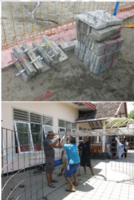
Figure 4: Medium and main structure.
