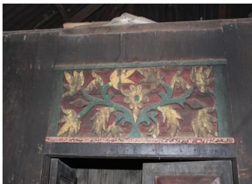
Figure 4: Malay House-Serdang Bedagai-2
