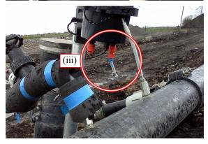
Figure 4: Site-specific issue rectification (i) Water-blockage, (ii) Tube shrinkage, (iii) Connection breakage due to pipe collapse.
