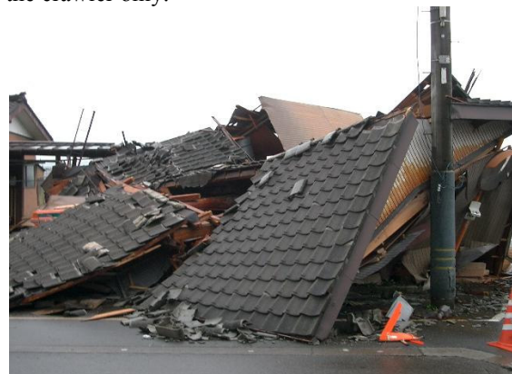
Figure 11: Collapsed Japanese-style house by Chu-etsu earthquake.
