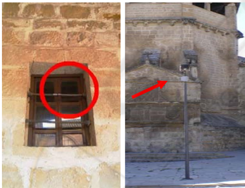
Figure 5: Examples of installations.
