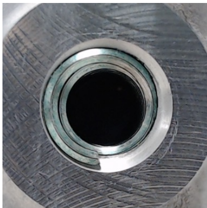
Figure 3: Example of a control area with a helicoil insert placed incorrectly (incorrect depth: too high).
