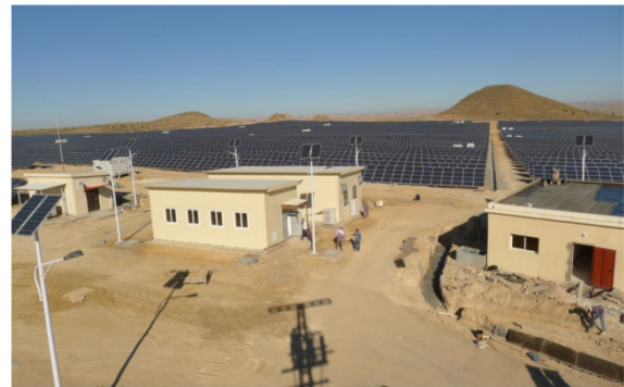
Figure 3: Photovoltaic Power Station of Oued Kebrtit.
