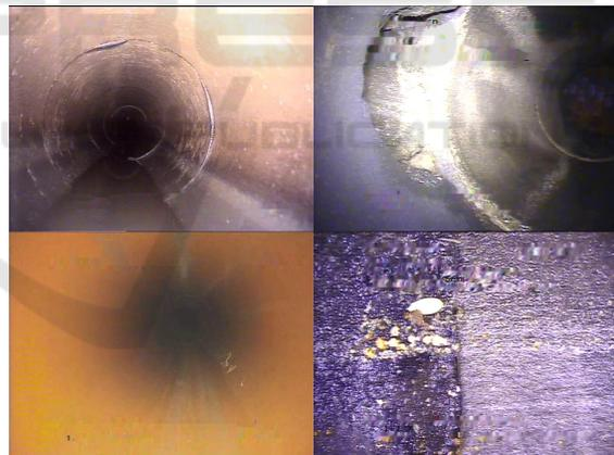
Figure 1: Challenging artefacts in real world sewer data.
