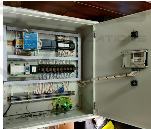
Figure 6: The control panel.
