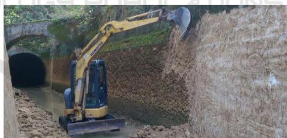
Figure 2: Removal of the tufa formed on the lateral sides of tunnel (URL 1).
