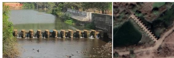
Figure 2: Photograph (left) and satellite image (right) of a gate based check-dam.
