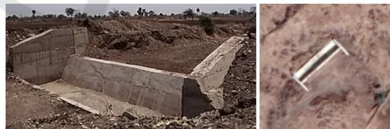
Figure 1: Photograph (left) and satellite image (right) of a wall based check-dam.
