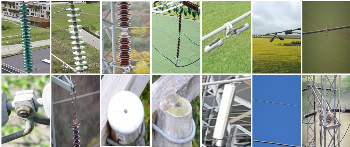
Figure 1: Sample images of normal and related most common faulty components classes used to train the DNNs model (from top left to the right bottom): Insulator type 1, Insulator type 2, Insulator type 3, damaged insulator, normal Vibration Dampener (VD), damaged VD, missing VD, normal Nutbolt, rusted Nutbolt, normal Toppads (Jenssen et al., 2018), missing Toppads (Jenssen et al., 2018), Antenna, broken Wire, Bird Nest, respectively.
