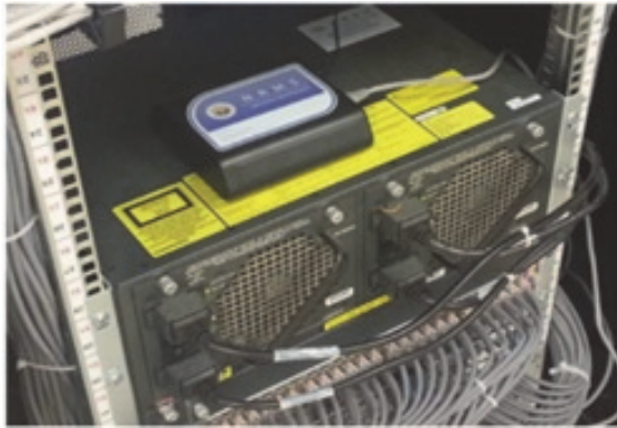
Figure 2: NRMS box connected to one of the servers.
