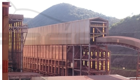
Figure 1: Example of storage silo from Brucutu mine – Vale.
