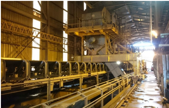
Figure 2: Example of tripper car from Brucutu mine – Vale.
