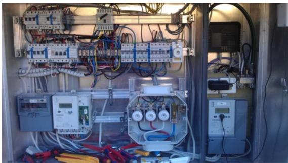
Figure 7: Real installation. The prosumer meter (top center) has been installed and wired in the existing electrical cabinet.
