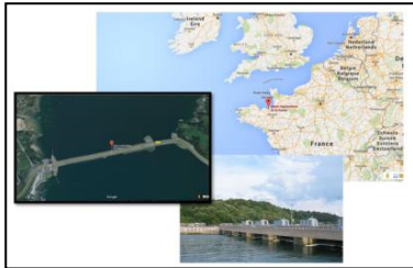
Figure 8: Location La Rance tidal power plant
