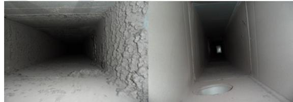
Figure 1: Before cleaning Air duct and After Cleaning.
