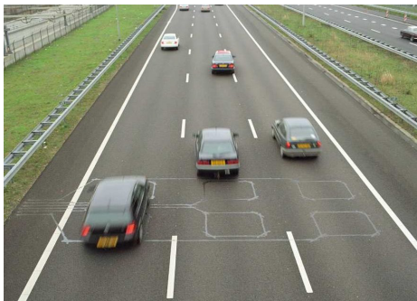
Figure 5: Wires in the surface of the road.
