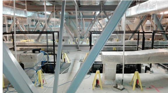
Figure 3: Sensor system with multi-point sampling in technical space.
