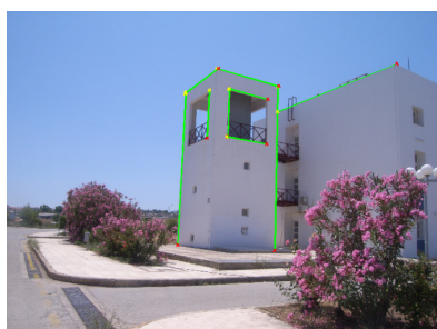
Figure 4: Lines belonging to the main structure of the target building and detected using the Hough transform. The yellow and red asterisks correspond to a line's beginning and end points respectively.
