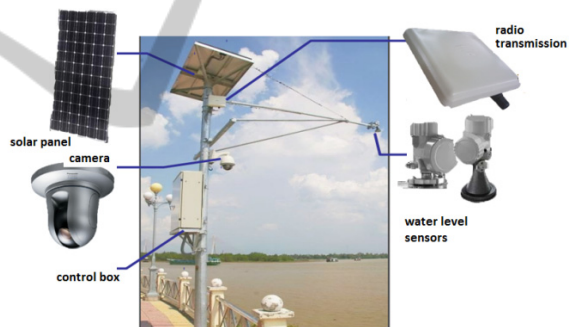
Figure 2: A fixed station for measuring water level of Can Tho city.
