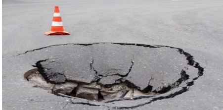
Figure 2: Condition of roads with potholes.
