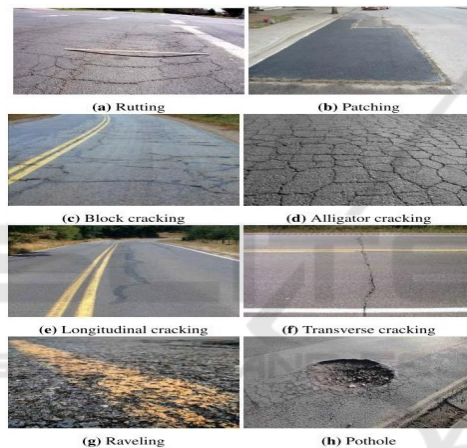
Figure 3: Road surface defects.
