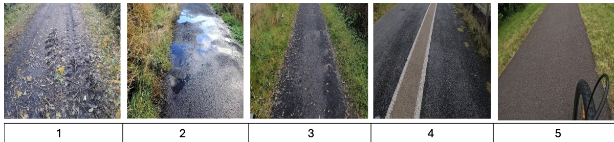
Figure 2: Sample image for each pavement condition rating: image 1-5 represents Rating 1 to rating 5.
