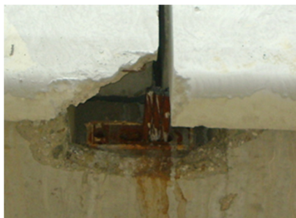
Figure 6: Un-grouted tendon duct.
