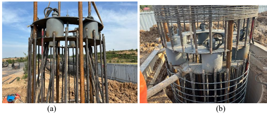
Figure 5: Installation (a) and welding (b) of steel cage.
