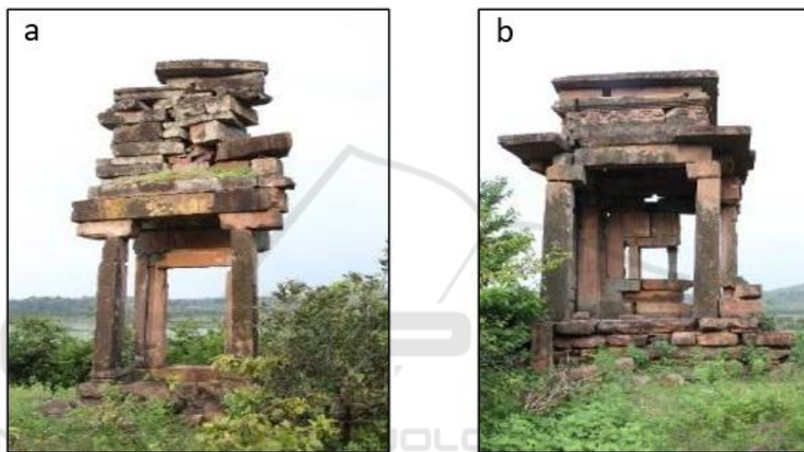
Figure 5: (a) &amp; (b) The Structures of 1st Site.
