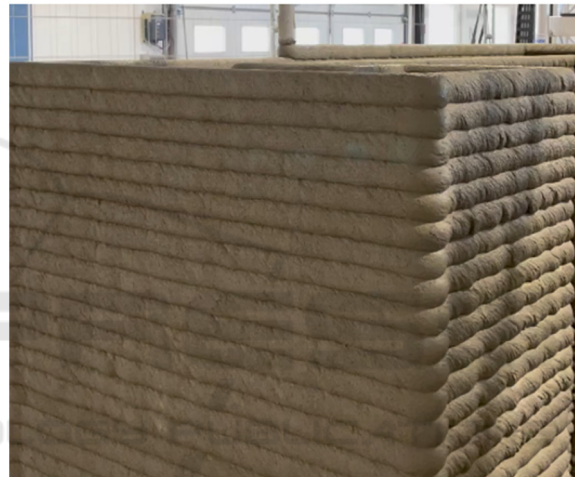
Figure 6: 3D Concrete Printing laboratory.
