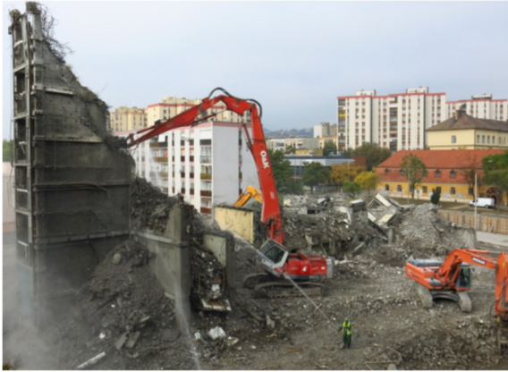
Figure 1: Demolition of High-Rise Building in Pécs, 2016.
