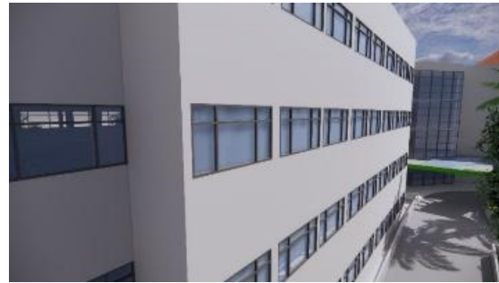
Figure 12: Existing Emergency Unit façade consist of walls, glasses window, and another opening.
