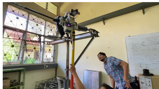
Figure 1: 20kV Shaft as robot hand operation tools.
