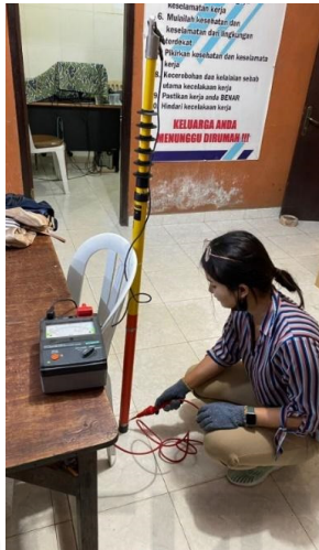
Figure 2: Dry insulation resistance test with Megger 10,000 Volt.
