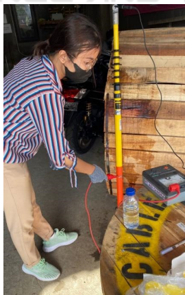
Figure 3: Wet insulation resistance test with Megger 10,000 Volt.
