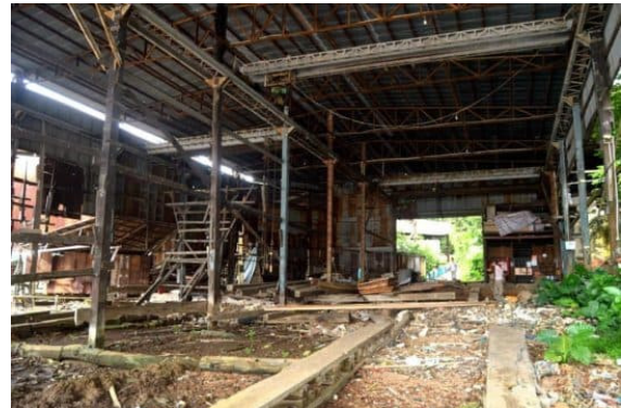
Figure 2: The history carried by the now abandoned Lai Chi Van Shipyard is gradually fading away.
