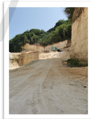
Figure 2: Excavation process in Melasti Beach.
