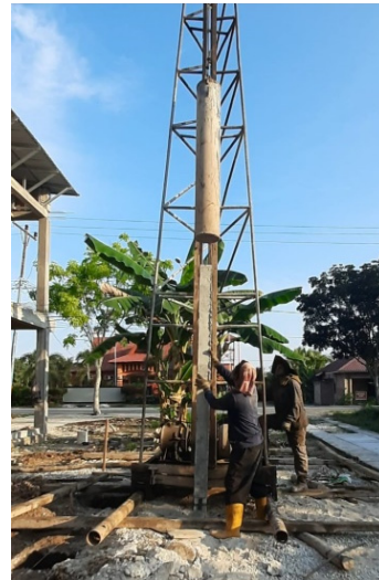
Figure 4: Erection of mini pile by drop hammer.
