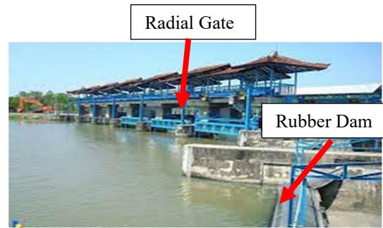
Figure 5: Radian Gate and Rubber Dam.
