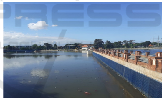
Figure 7: Bar Screen and Groundsill.
