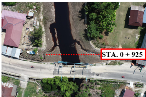
Figure 5: Research locations STA 0+925.
