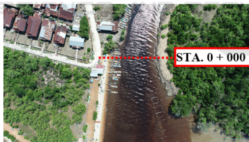
Figure 4: Research locations STA 0+000.
