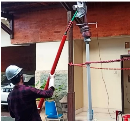
Figure 5: Online pedestal insulator washing.
