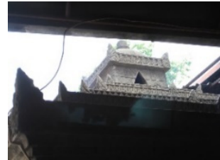
Figure 57: Roof of Siti Moyo.
