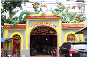
Figure 53: Front gate of Klenteng Hong San Ko Tee.
