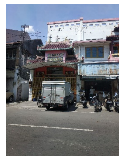
Figure 52: Front view of shophouse at Kembang Jepun.
