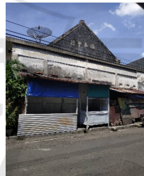
Figure 51: Front view of shophouse at Kembang Jepun.
