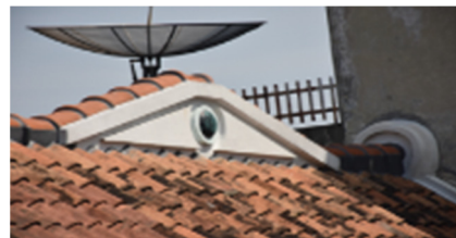
Figure 8: Additional ornaments were added during the late Mr. Lin's father, intended as Chinese geomancy (feng shui) elements against bad things (sha qi 杀气).
