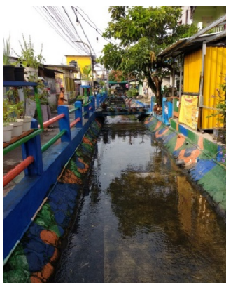
Figure 2: Open Space an Circulation Along Babakan Irigasi Stream.
