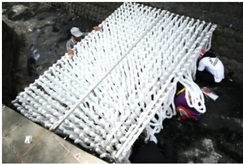
Figure 6: Bio-Cord Installation at Cikapayang River.
