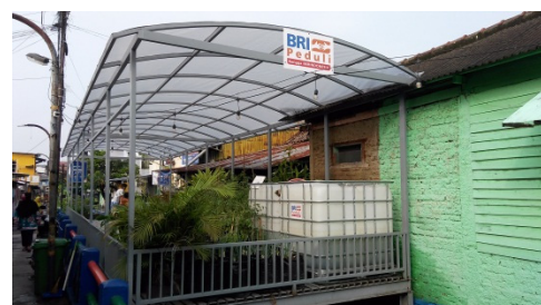
Figure 15: Clean Water Ground Tank Reservoir.
