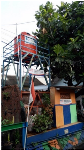
Figure 16: Clean Water Upper Tank Reservoir.
