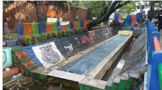
Figure 8: Bio-Cord Installation at Babakan Irigasi.
