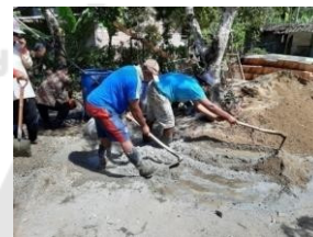
Figure 1: Imperfect concrete manufacture.
