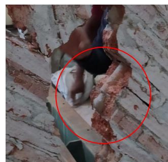
Figure 18: PLB brick-shaped mortar pegs.
