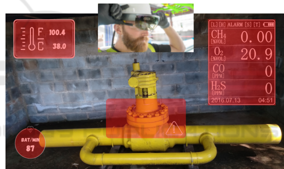
Figure 2: Using augmented reality to visualize sensed information in the confined space. Operator using Trimble Connect and Microsoft HoloLens. Source: Author, adapted from (Trimble, 2021).
