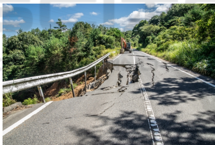
Figure 2: Road collapse site.
