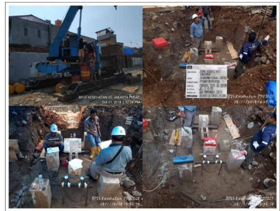
Figure 2: Piling and instalation of PDA test.
