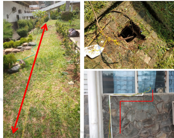
Figure 1. Ground Mesh Location and Wiring
