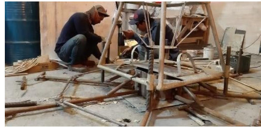
Figure 3: web frame of ADP construction.
